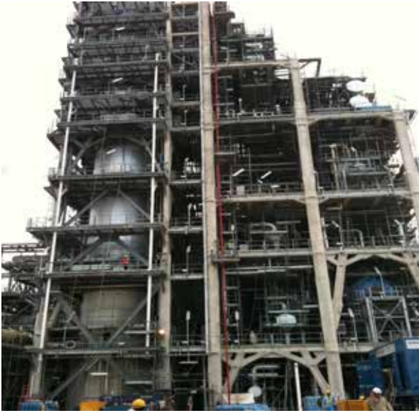
Equipment Skirt & Steel Structure Fire Proofing
